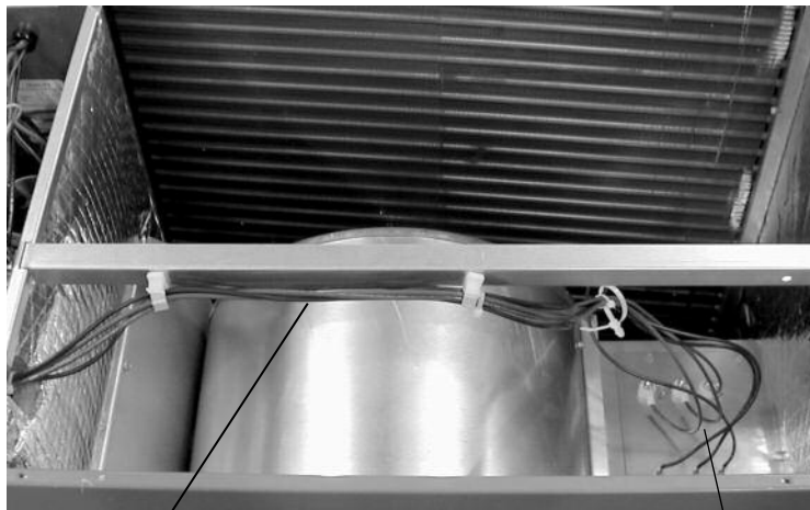
FIGURE 5 HEATER KIT INSTALLATION
